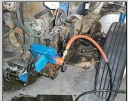
DK50 Hydro-Clamp Repair
